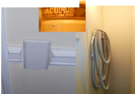
Dual central vacuum system makes cleaning easy and convenient. Vacuum ports are located in all apartments, hallways, and in the lobby area.
